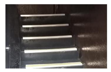
The hall stairs in Avondale House have been fitted with a non-slip surface with metal lips to provide safer access for residents.
