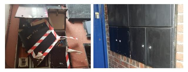
Four sets of Utility Boxes at the front entrances of O'Brien Hall which had been vandalized have been repaired removing the danger of exposed electrical cables to residents.
