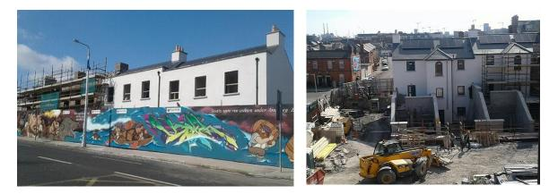
External rendering has been completed on Nos. 2 - 4. No. 5, the construction of which was delayed, is now on stream with the external walls completed and the tiling of the roof underway. Current completion date for the entire complex is summer 2019.
